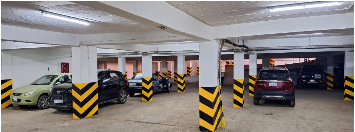
Picture 2: Basement upgrading work
