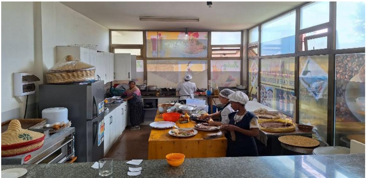
Picture 1: Cafeteria kitchen upgrading works
