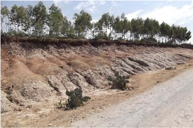
Figure 4: Roadside soil erosion, Boricha district, February 22012 © S. Hameso
